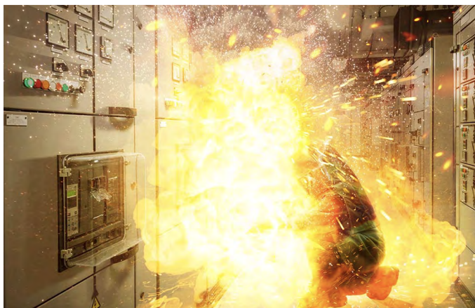
Figure 4-4. The dangers of arc flash can not be understated.
